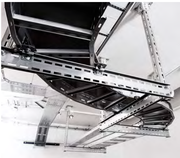
Bolted support system with shared support between disciplines. Flexible for future changes of the installation.
