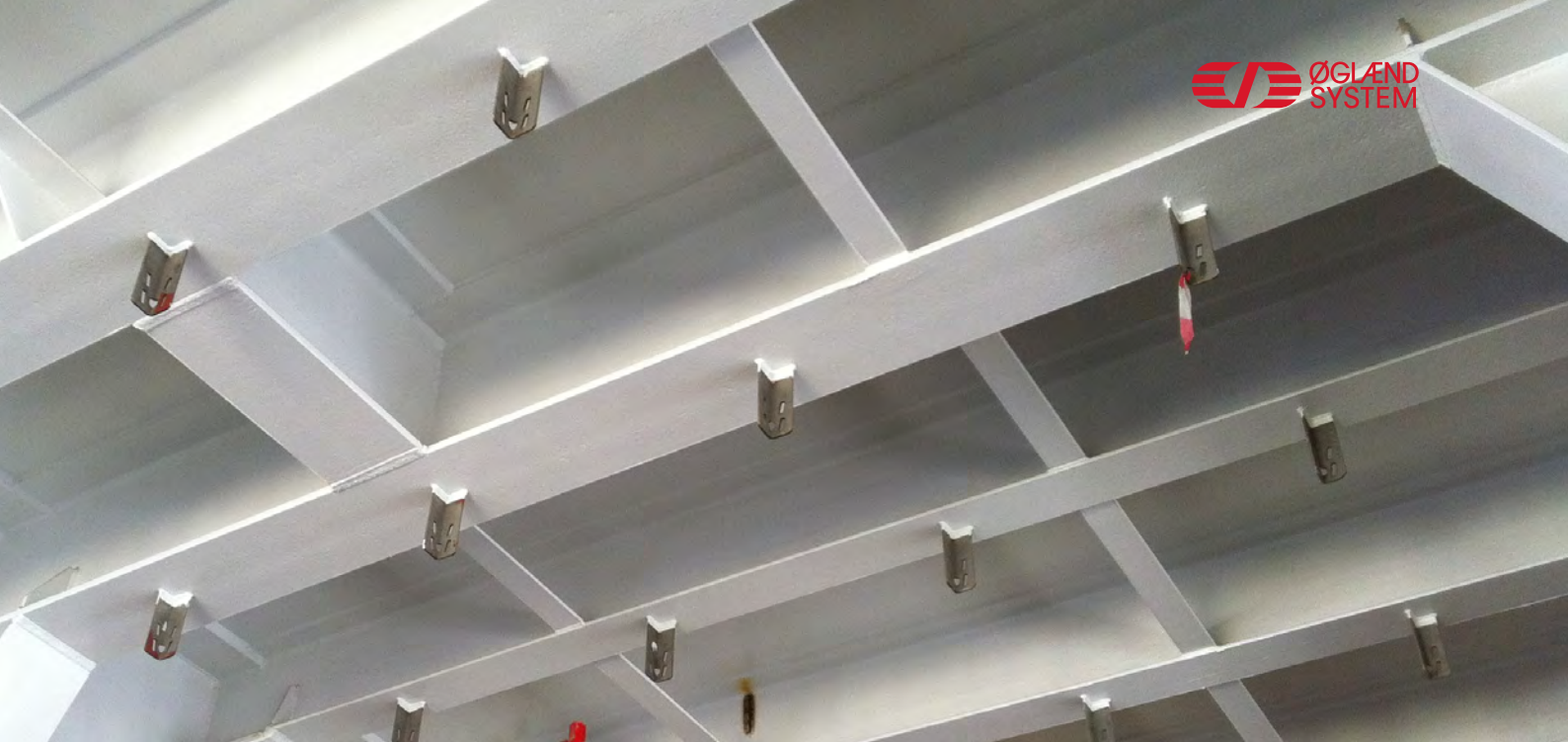
MultiGrid® installation concept - starter brackets welded to structure in a grid pattern for full flexibility.
