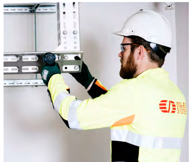
Bolted support system with shared support between disciplines. Flexible for future changes of the installation.
